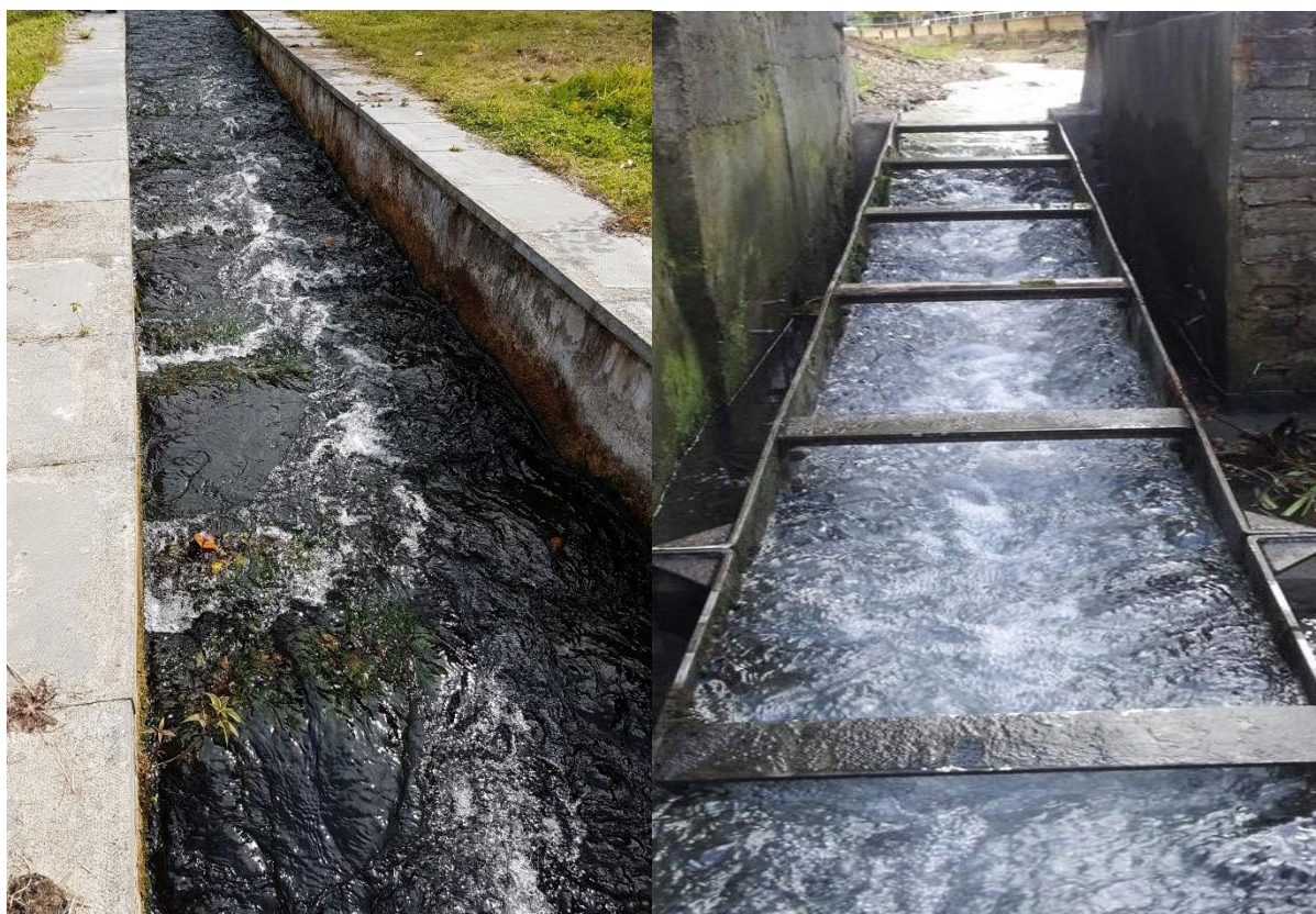
Figures 8 & 9. Examples of a Hassinger bristle pass (left) and a Larinier superactive baffle fish pass on the Wandle at Carshalton (right).
