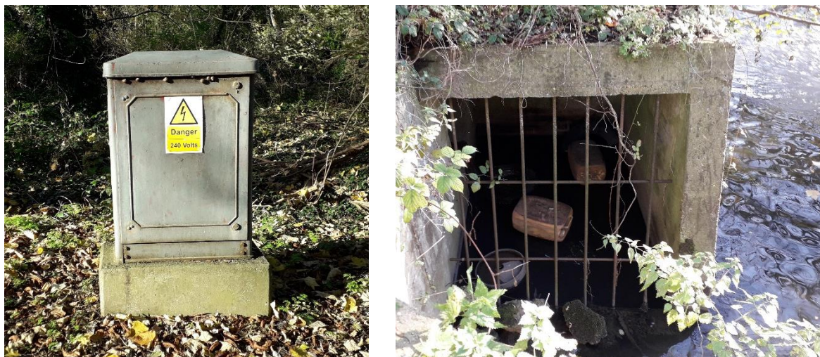
Figure 3. Photos of know utilities not highlighted by desk based utility search.
