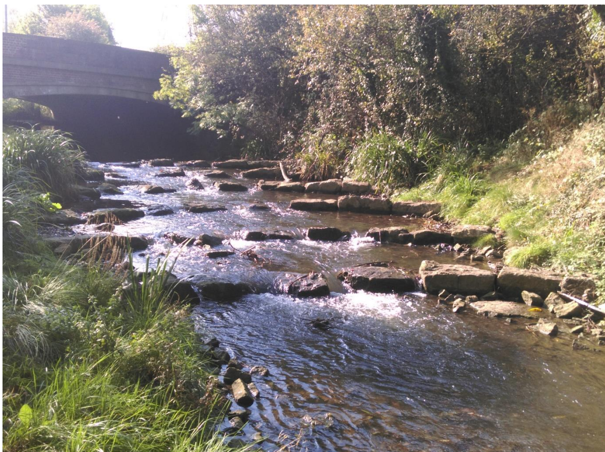
Figure 6. Rock ramp structure on the Hogsmill River near Kingston, London.
