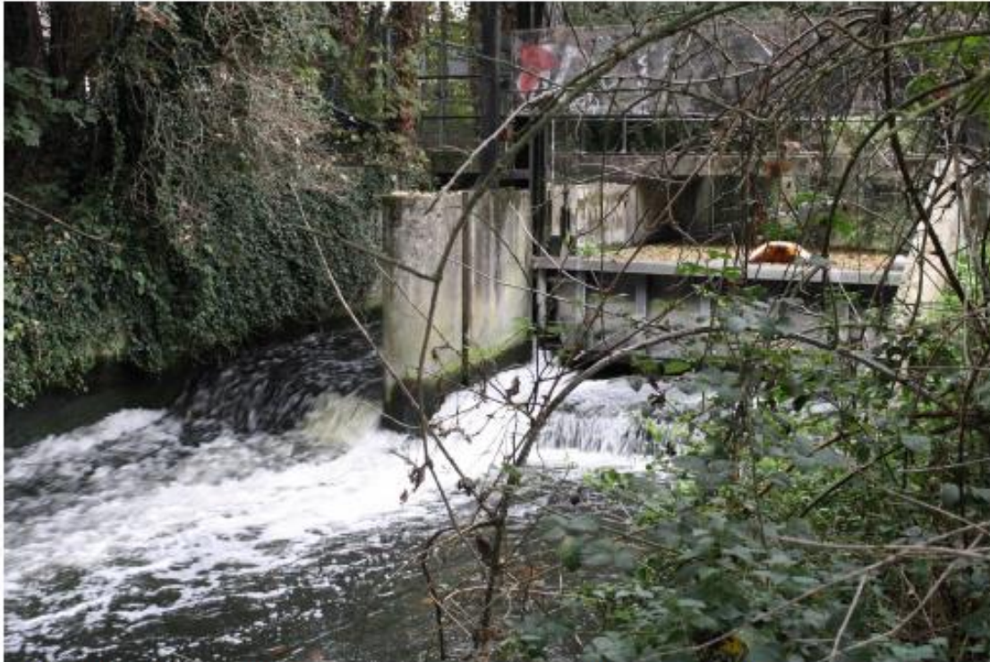
Figure 5.18. Undershot sluice at Watermeads Weir. The outfall from the sloping channel (Figure 5.20) can be seen on the left of the picture.
