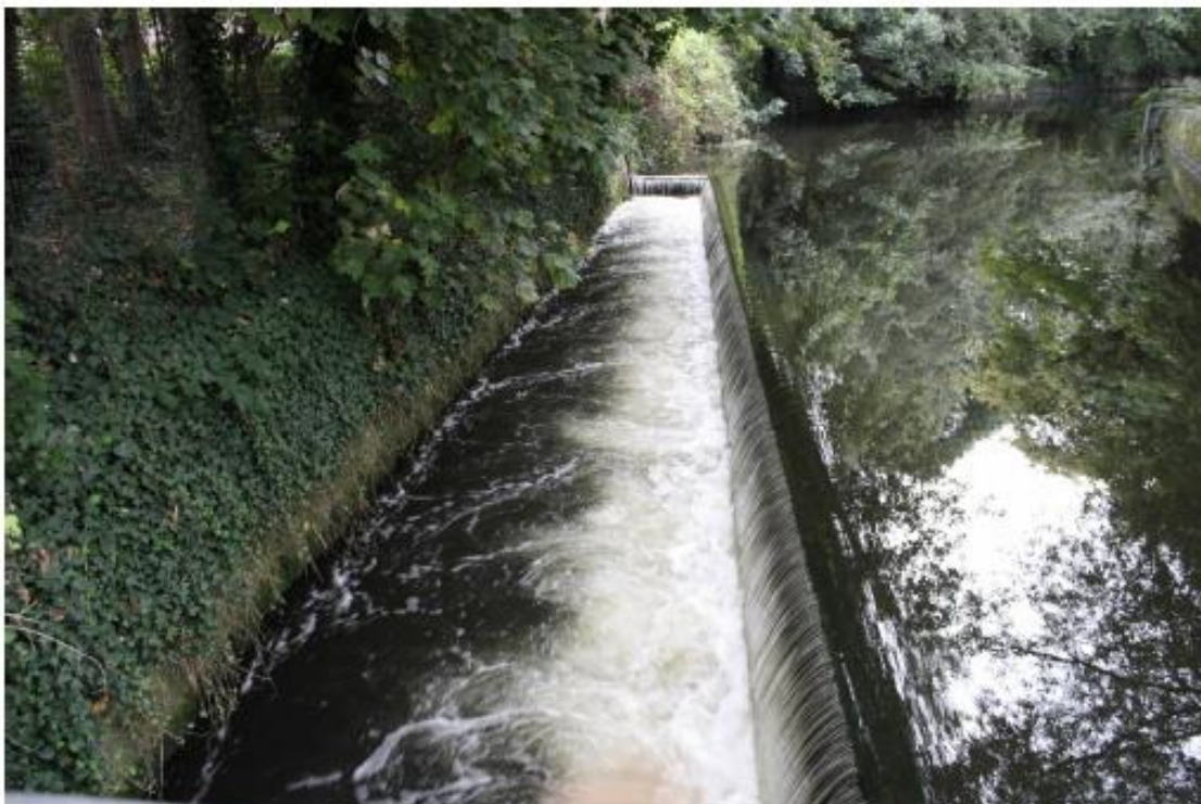
Figure 5.19. Sloping channel fed by long-crested weir, Watermeads.
