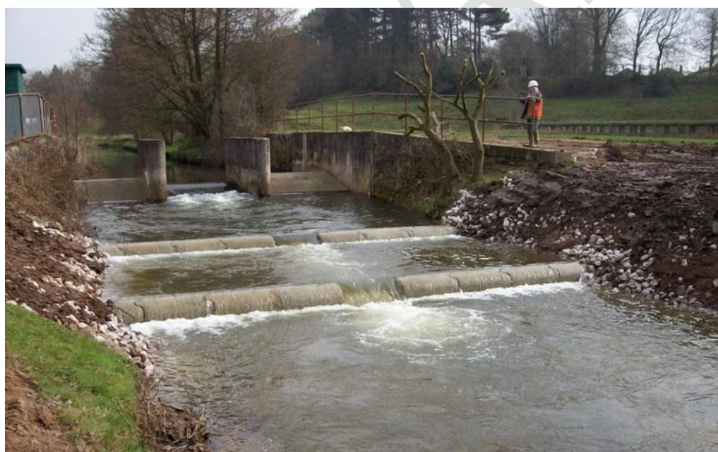
Figure 5: An example of a pre barrage used by Environment Agency to ‘drown out’ a weir - CT Construction Ltd.
