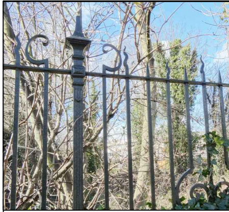
Existing bespoke railings on Mitchum bridge
