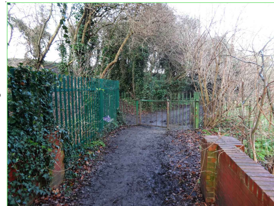
Photo 2: Existing entrance :Brick walls to be retained part of flood defence, green palisade fence to be removed
