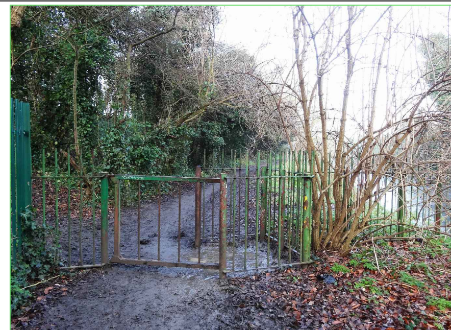
Photo 1: Existing vertical rail with kissing gate: To be removed
