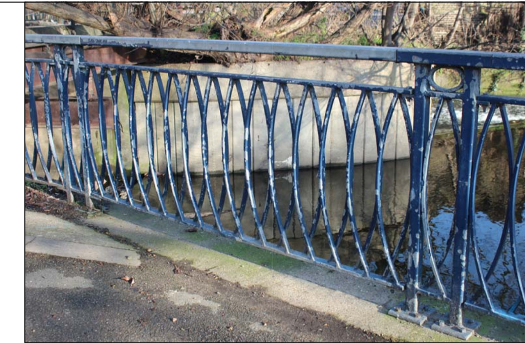
Existing riverside railings
