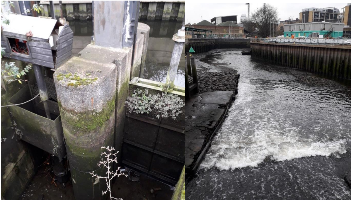
Figure 3. Bell Lane sluice. Double penstock structure (left) and the Bell Lane creek below the structure, which includes a long concrete apron (right).
