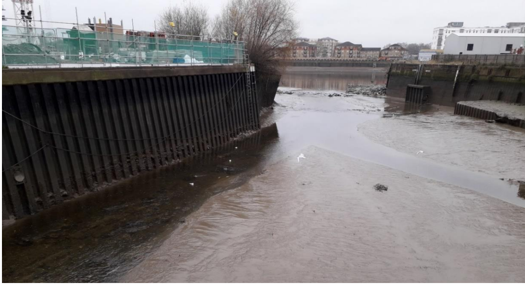
Figure 5. The downstream confluence of the bifurcated channels below EDF weir and Bell Lane sluice at low tide. Flow from the EDF structure joins from the right-hand-side and flow from the Bell Lane sluice joins from the left-hand-side. There appears to be a greater proportion of freshwater flow joining from the Bell Lane sluice structure, giving this structure a better attraction flow for migrating fish under the current flow split.
