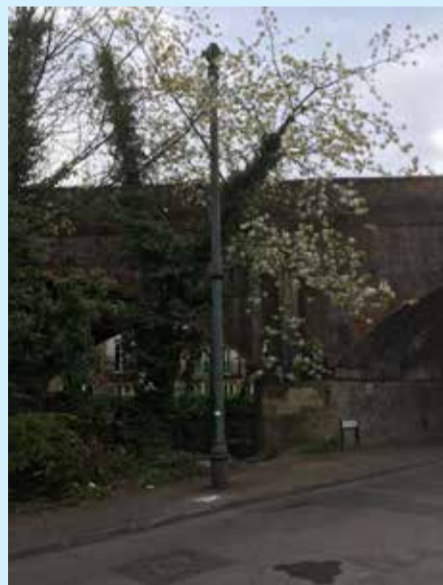
A stench pipe – just one of the many existing clues to look for!
