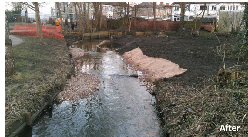
Figure 2: Ravensbury Park Before and After Photos
