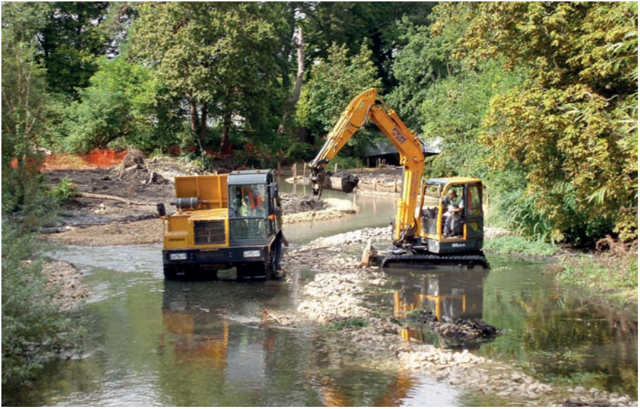
Re-profiling the river at Hackbridge – September 2014.
