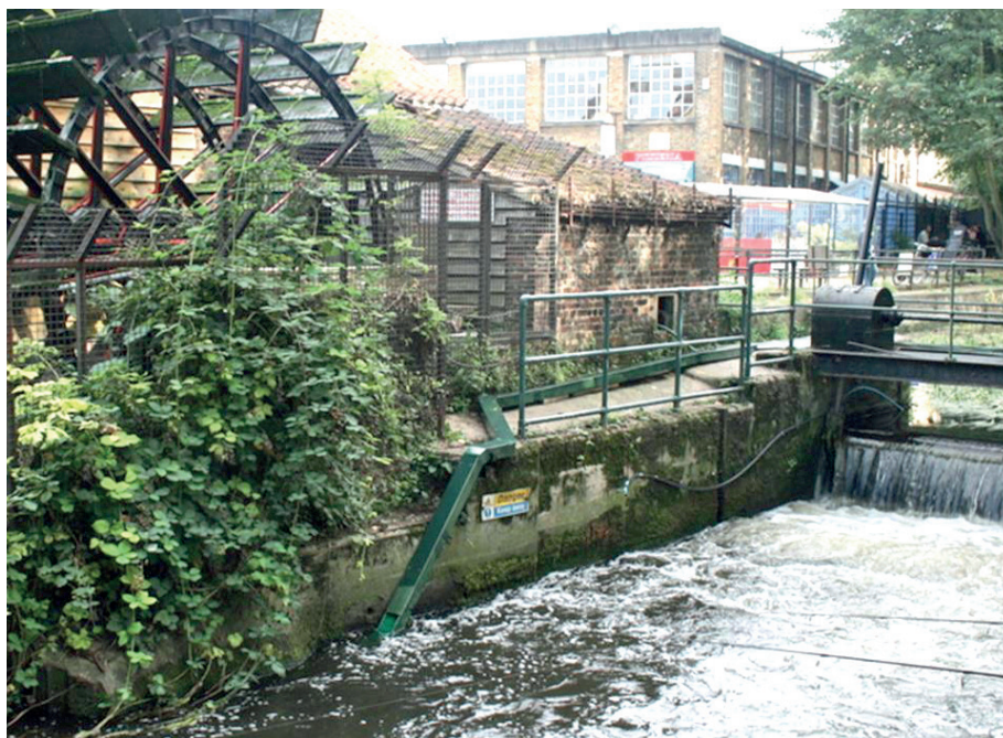
Merton Abbey Mill, weir and eel pass.
