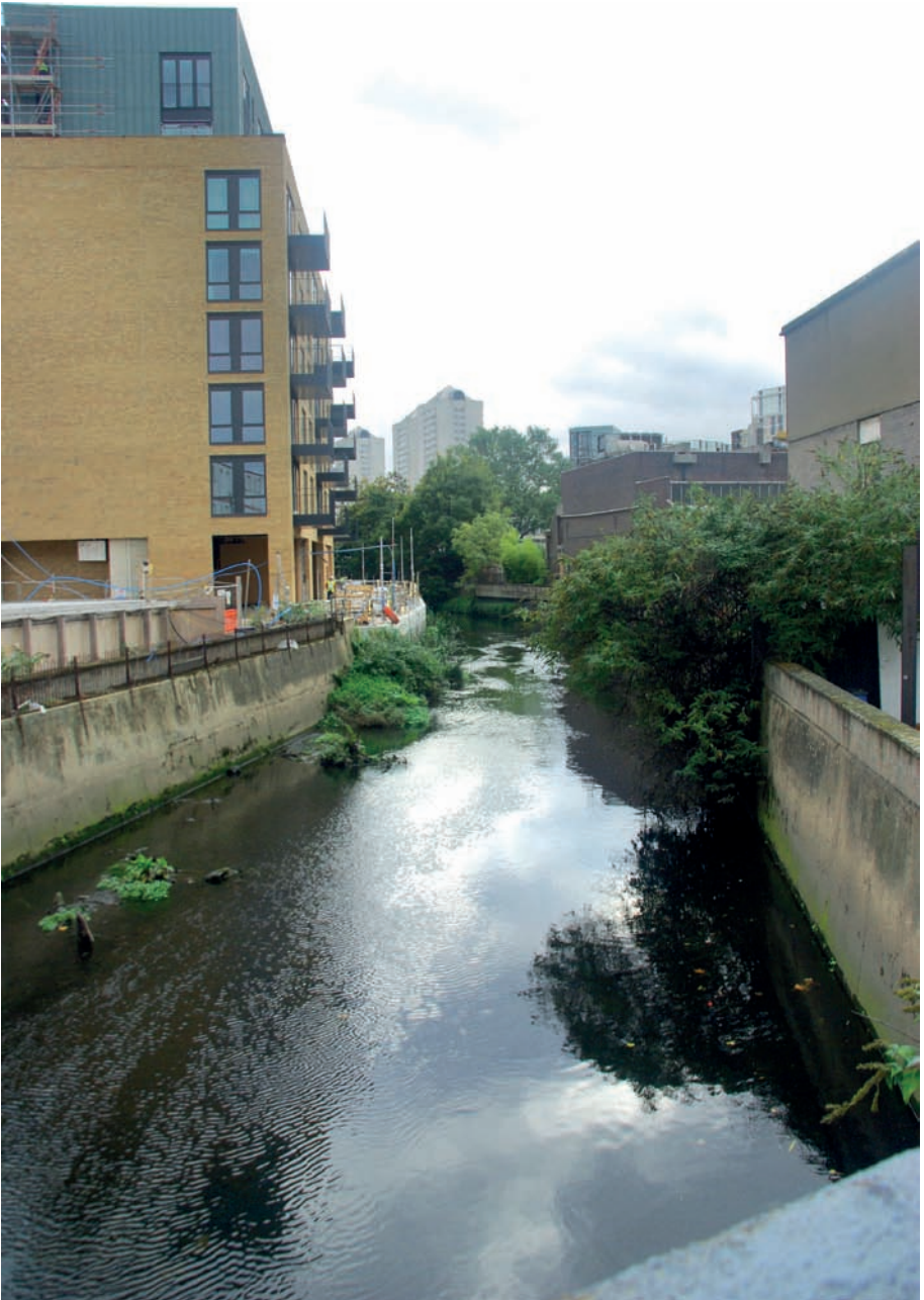
Looking upstream into the Ram Quarter.
