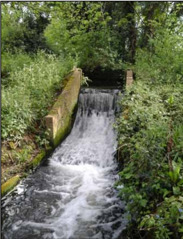
End support to Snuff Mill Waterwheel Image Courtesy of: Stuart Swan
